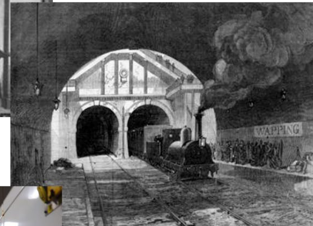
In 1860 was converted into a railway tunnel for the East London Line, later absorbed into the London Underground.
